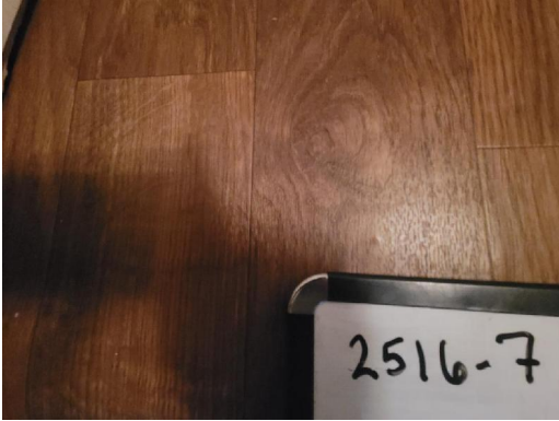
2516-7 Rolled Flooring/Mastic Interior Bathroom
