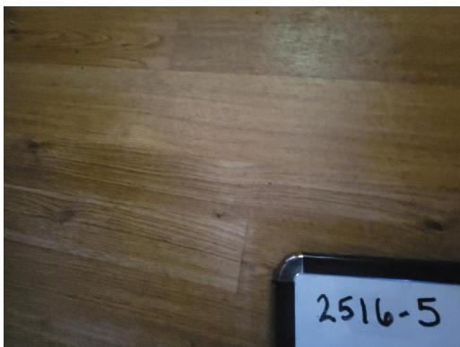
2516-5 Rolled Flooring/Mastic Interior Kitchen
