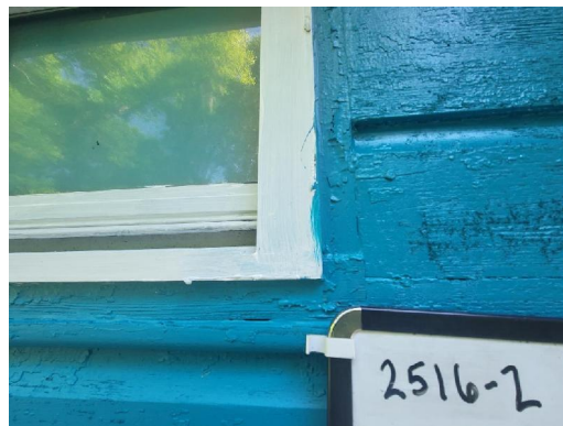
2516-2 Caulk Typical Exterior Windows
