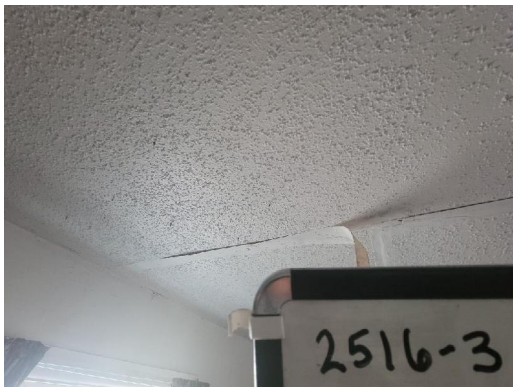
2516-3 Popcorn Ceiling Texture Interior Living Room/Bedrooms
