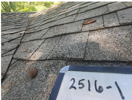
2516-1 Asphalt Shingle/Tar Typical Exterior Roof
